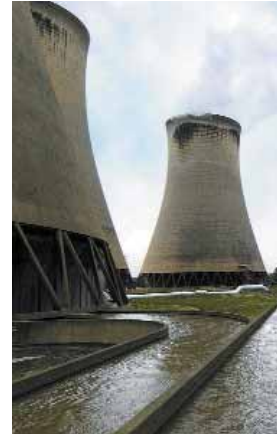
Cooling towers at Drax Power Station
